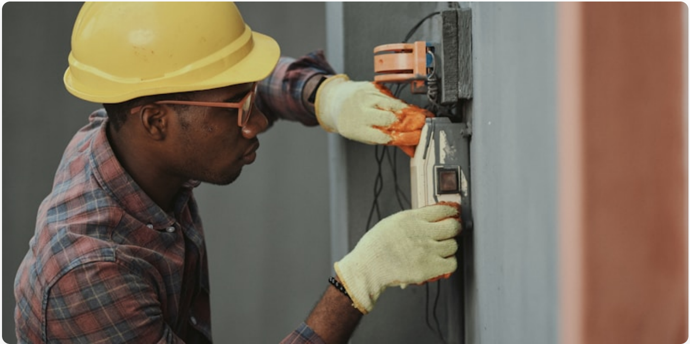
Figure 3: 2026 Fire & Life Safety Industry Report highlighting new compliance requirements
